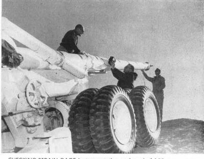
CHECKING STRAIN GAGE instrumentation on barrel of 155 mm gun are Ed Healy, Art Thomas, and Jim Shindelar, all of 8121-4. The gages, placed two-feet apart along the length of the barrel, will obtain data on the acceleration of projectiles fired through the cannon barrel.
